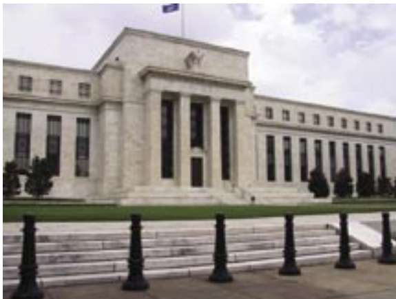
The Federal Reserve Building, Washington, D. C.
