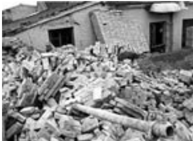
Damage to the Fushan Christian Church after the mob attack. (Fushan Christian Church photo via ChinaAid).
